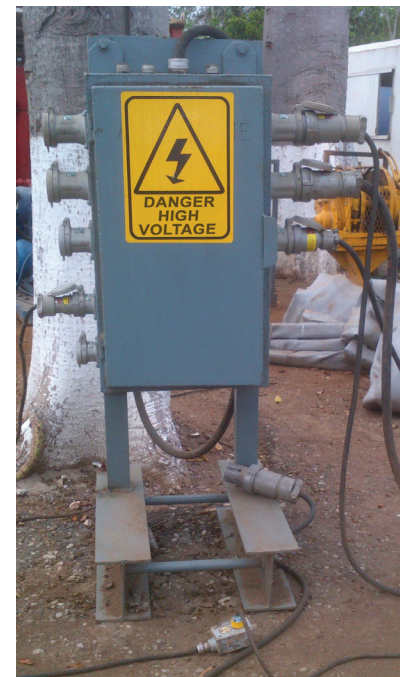
Appleton Powertite Plugs and Receptacles - providing power to pumps and compressors.
