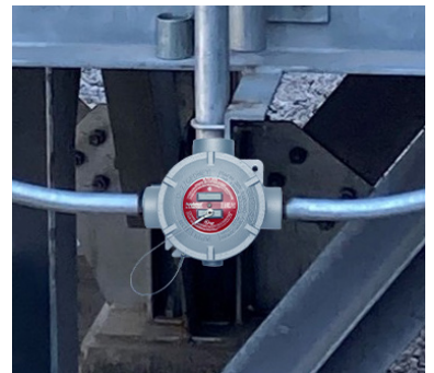
Stanchion mounted lighting at a natural gas facility
