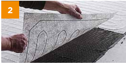
Lay down Warm Tiles™ Elite mat.
