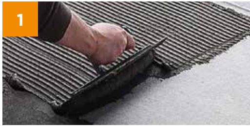
Apply thin layer of mortar to floor.
