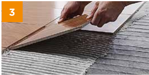
Apply thin set and install floor surface.
